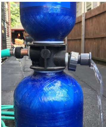
Figure 10: Whole house water filtration system with reduced water flow, possibly due to phosphate-based corrosion inhibitor.
