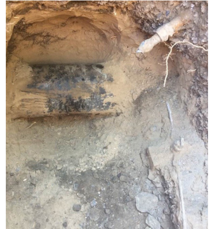
Figure 5: Circa 1890 Humboldt Parkway water main. Note the 3/4" copper service on the bottom right and the older 1/2" disconnected lead service at the top right.
